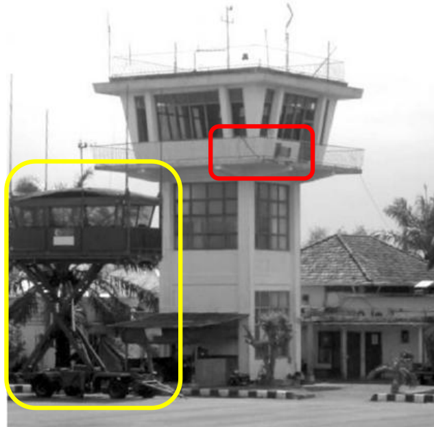
Figure 2.2. Cracking in the Control Tower and Portable Control Tower at Banda Aceh Airport 3
